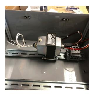
4) Connect the 50VA Potential Transformer to the same DIN rail as the terminal block. Orient the primary side (colored wires) toward the terminal block. The black wire on the primary side of the transformer is the neutral line. Important: Ensure that the neutral line of the transformer connects to the same block as the neutral line of the incoming distribution panel!
